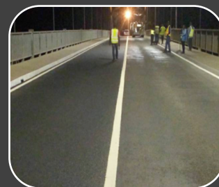
Night work to eliminate traffic issues
