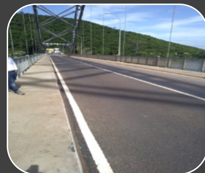
Nov 2019 - Resealed bridge
