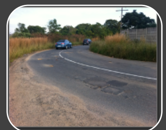
2015 – after 17 years the wearing course is brittle and showing severe signs of wear. However, the stabilized base layer is still intact with no rutting or deformation
